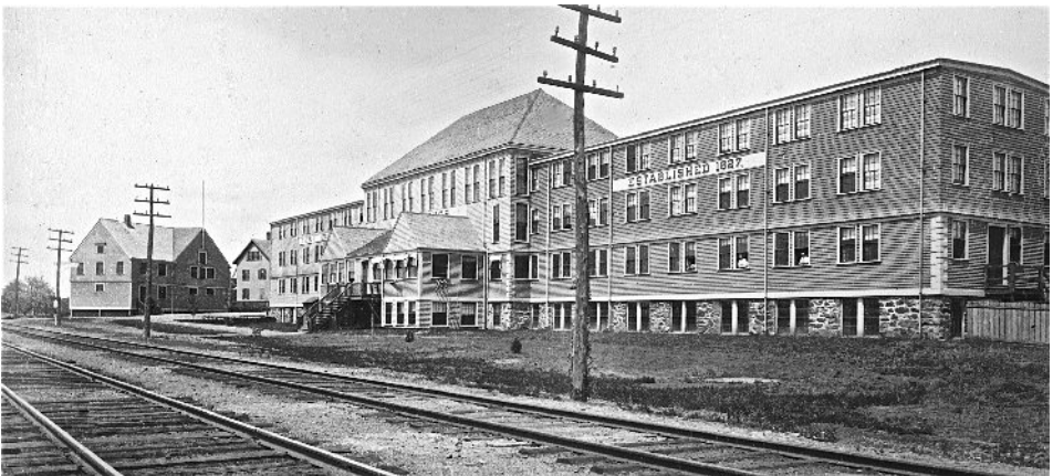
Fire was of particular concern for organ factory owner Francis Henry Hastings, whose 280-foot-long, wood-frame factory building was located next to the railroad tracks on Viles Street. Burning embers from trains were a common cause of fires. The Hook & Hastings Co. purchased Weston's first fire truck and donated it to the town. (WHS photo)
