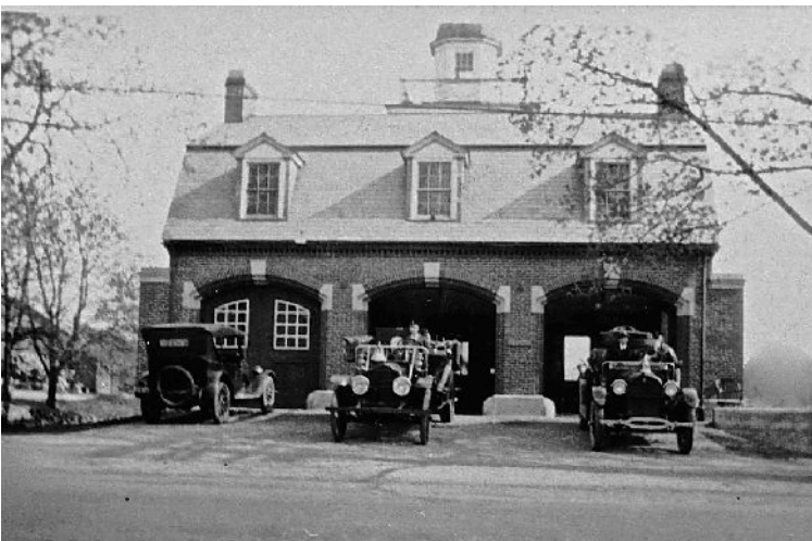
This c. 1920s photograph shows the new fire station with its original doors and two early motorized fire-trucks. (Courtesy Beverly Historical Society Walker Collection)
