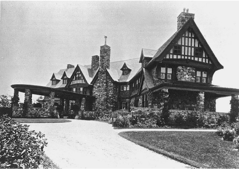
This elegant Tudor mansion on Westcliff Road, built for Arthur Clapp, was purchased by Boston wool merchant Edward R. Peirce in 1909. It was destroyed by fire in 1925 and rebuilt in similar style using almost the same floor plan. The second mansion is now known as Henderson House. (WHS photo)
