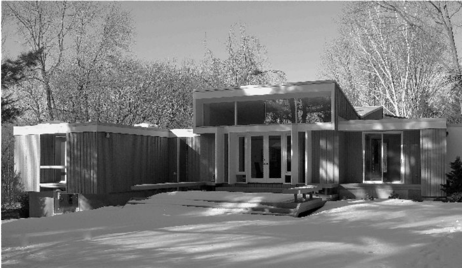
Above: Floor plan and section of the Kurt Fuchs House, 460 Conant Road (From Record Houses of 1968) Below: 2010 photo of the Fuchs House by Pam Fox.
