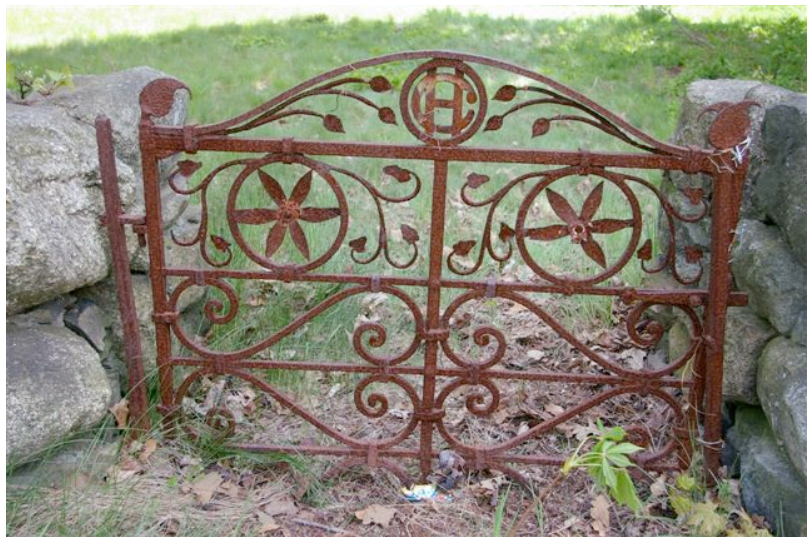
The Hillcrest logo, an interlaced H-C, is seen on this iron gate along Wellesley Street. It was probably made by Weston blacksmith Oliver Patriquin, who made ironwork items for many local estates.
