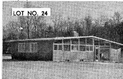
THE DAIRIKI HOUSE
