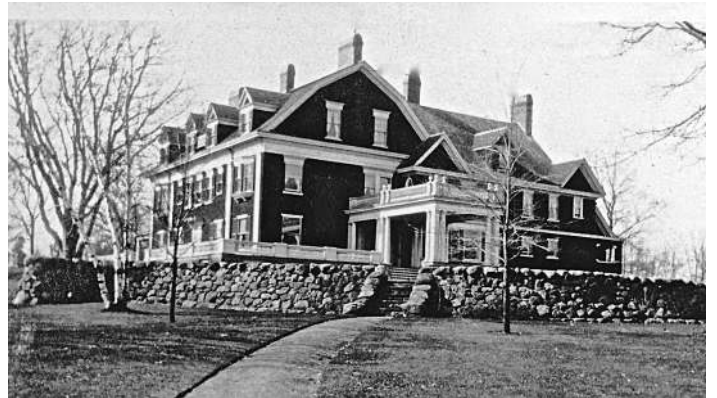
The Charles Dean estate mansion at 67 Byron Road (above) was demolished in 1961.
