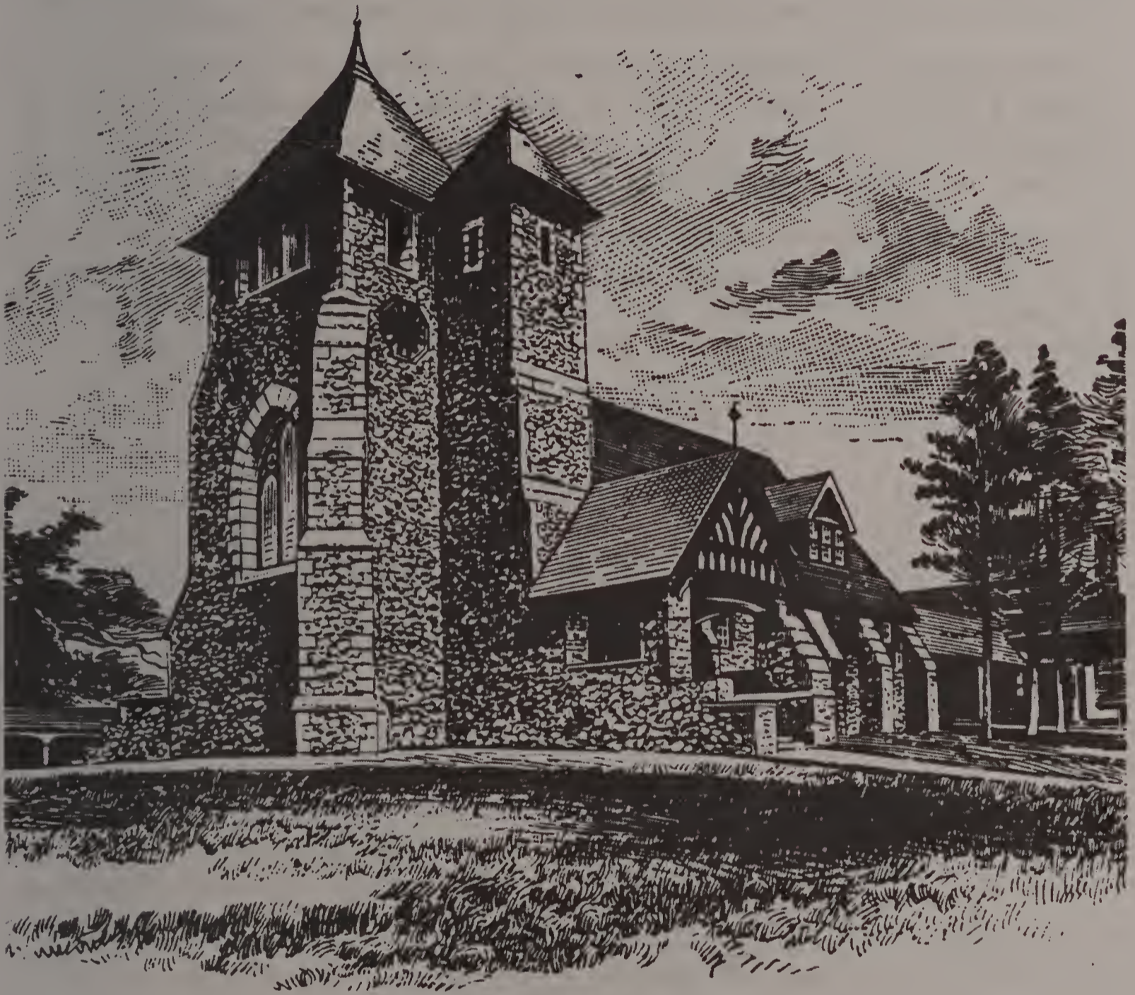
The 1888 First Parish Church.
