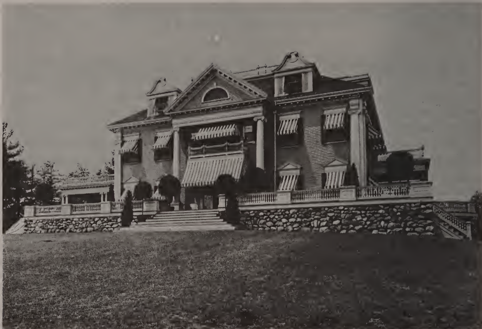
The original Demmon-Morrison House: notice the clapboards.
