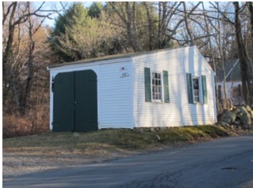
During the Depression, Oliver Patriquin moved his blacksmith shop from the town center to this small building at the corner of Love Lane and Boston Post Road. (Photo by Pamela Fox)
