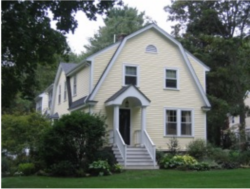
40 Chestnut Street (above) and the three houses behind it were built on Oliver Patriquin's land. No. 40 was constructed about 1920 by carpenter William Henderson, who lived down the street. It was remodeled in the early 2000s. (post-renovation photo by Pamela Fox)
