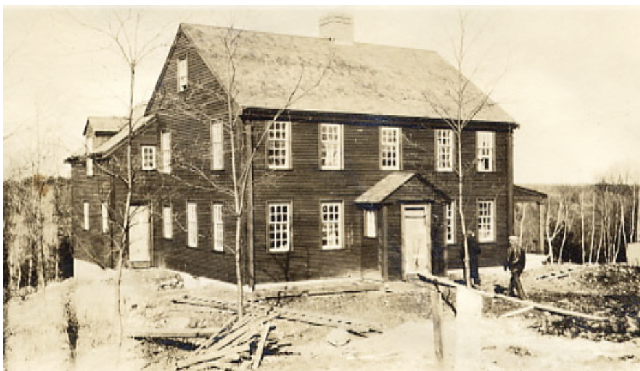
Author William Howell grew up at 326 Highland Street. This 1929 photograph shows the house as construction was almost completed. (Photo courtesy of Wm. Howell)
